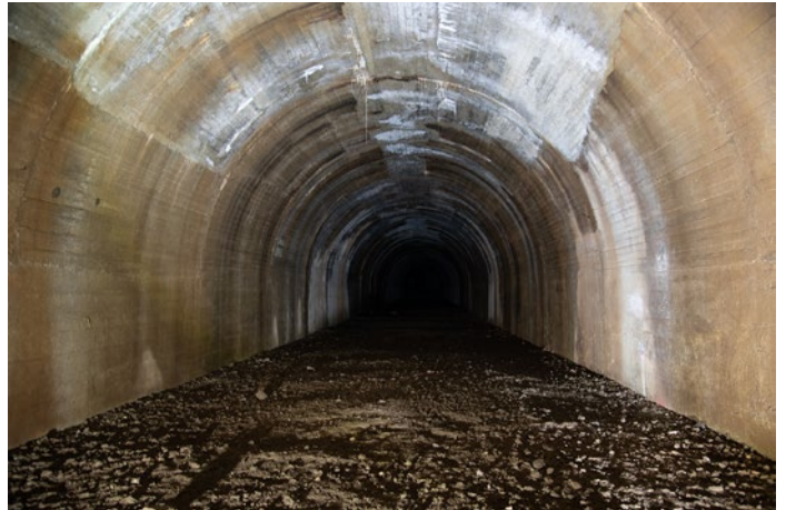
(Fig. 3) A section of the Galleria Rifugio photographed before the reopening process and redevelopment works began.
