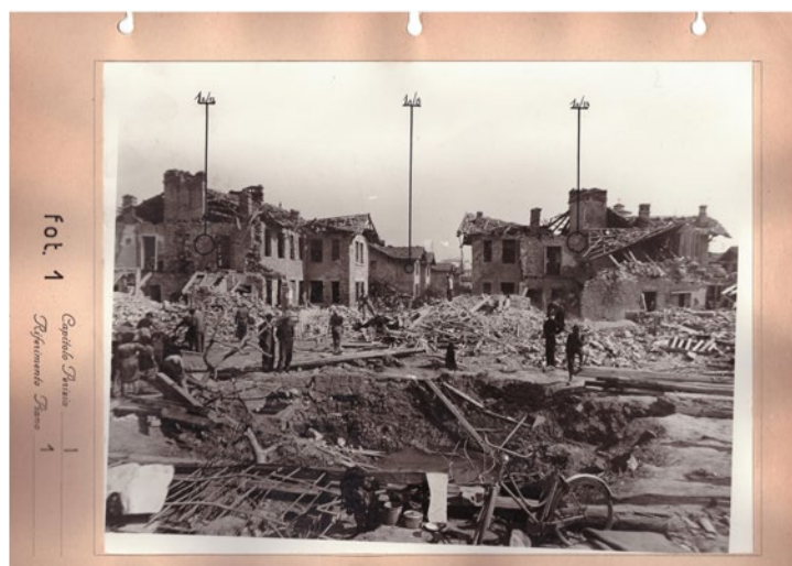
The working-class district of Panzano after the bombing in the spring of 1944. Photo: Francesco Penco, 'War Damage' report, Associazione Edile di Pubblica Utilità Monfalcone (Public Utility Building Association of Monfalcone), 1944. Private Coll. Pietro Commisso.
